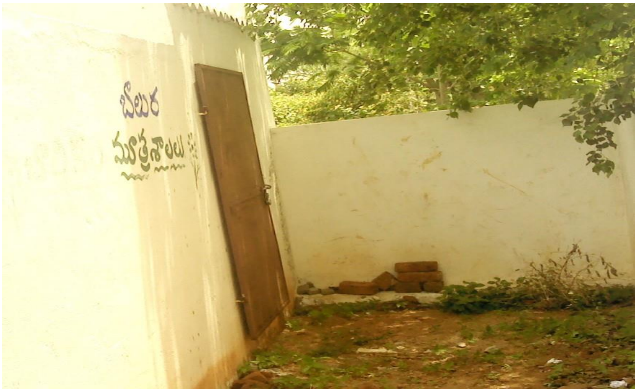
Toilets constructed but locked due to without water in Chinnakodur, Medak district
