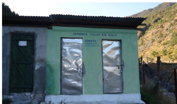
Well constructed toilet
