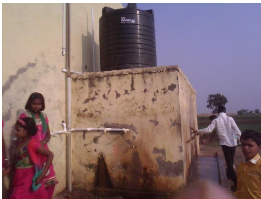
(Drinking water facility at school)
