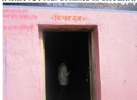
(Picture :4 Kitchen Shed available but not in use)
